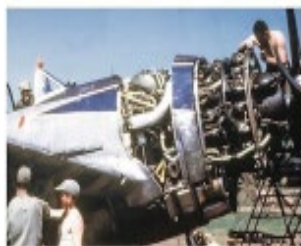
Center left and right: Two additional vintage color photographs of mechanics working on the huge Pratt & Whitney radial provide a good look at its details. Note the rounded conical shape of the reduction gear housing with the magneto on top of it. This early Thunderbolt has the original Curtiss Electric propeller installed. (Both, Bell Collection)
