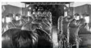
The interior of the C-87 had seating for as many as twenty-five passengers. The seats could be removed to carry up to 12,000 pounds of cargo. (Lloyd Collection)
